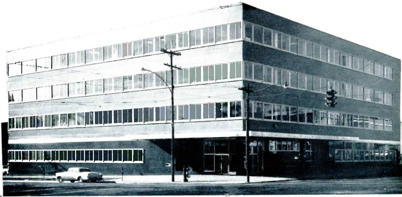
This modern office building in Salt Lake City houses the general offices of Mountain Fuel Supply Company.
