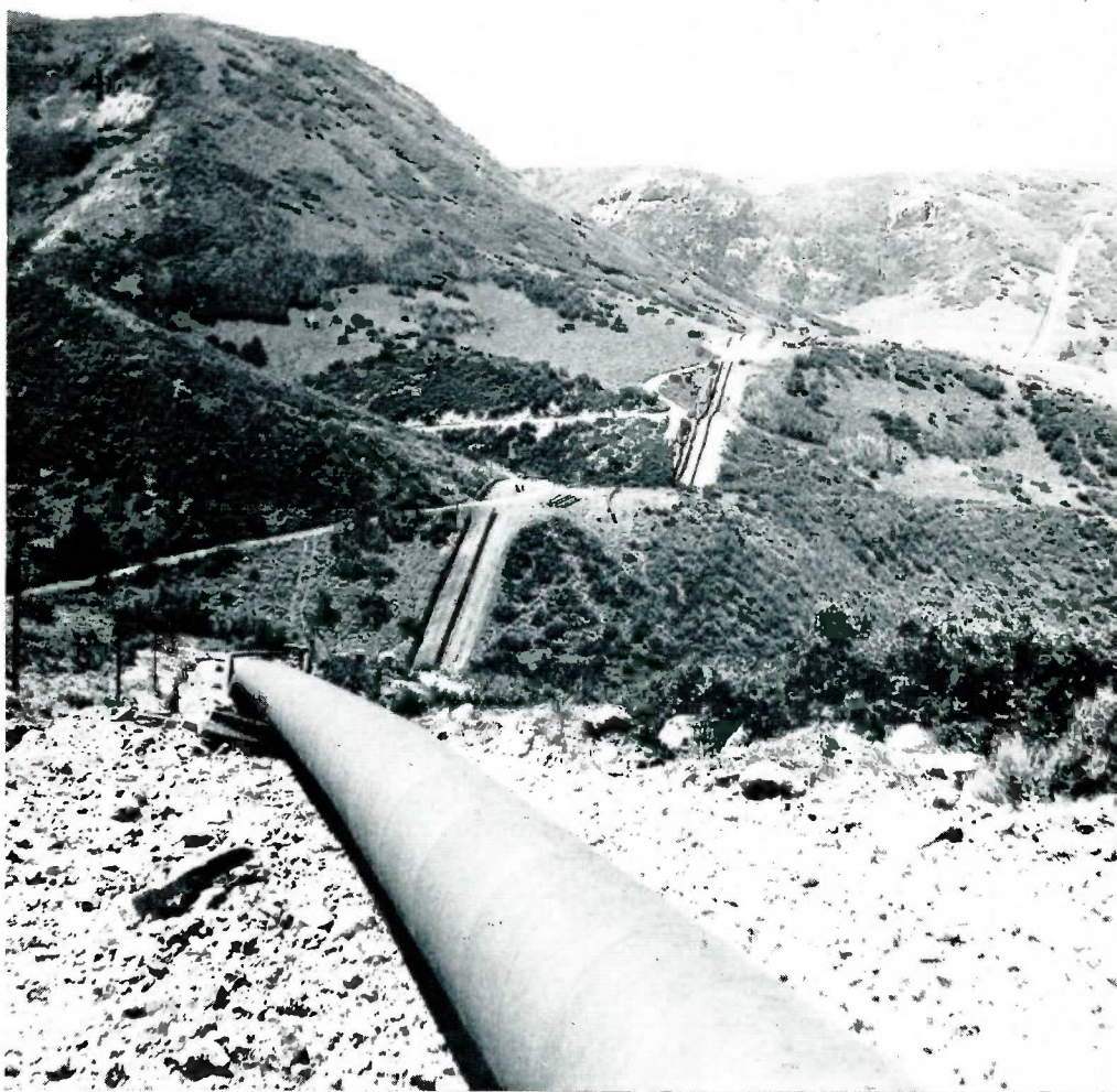
East of Salt Lake City, a 24-inch natural gas pipeline was installed in 1963 to replace a 16-inch line originally installed in 1929 for Mountain Fuel Supply Co.
