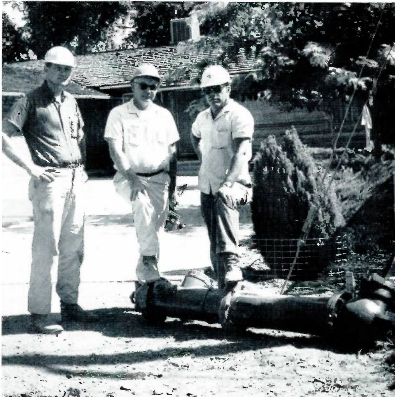
Kirkwood-Bly Inc., of Santa Rosa, Calif., installed 25 miles of distribution main for the project. From the contracting firm are, from left: Cass Bly, Jim Kirkwood and Bud Bartram.
