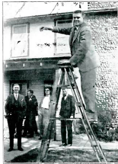
Billy Jett giving an exhibition of the proper way to wash a window before placing a Mueller exhibit
