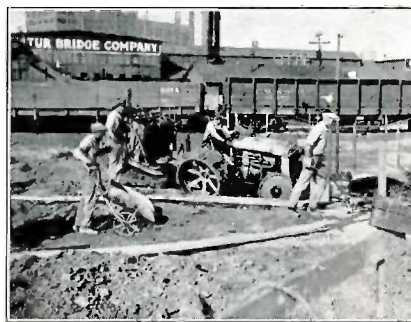
Leveling up for the foundation for the new iron castings department
