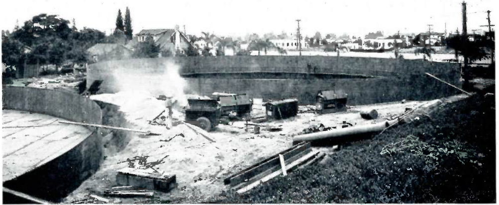
Construction scene at Alhambra where two large reservoirs were installed.
