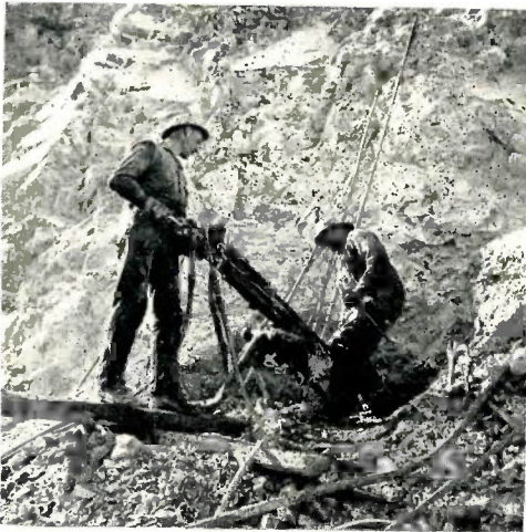
Drilling blast holes with a rock drilling machine at the open-pit mining operations of the Utah Copper Co., at Bingham canyon.
