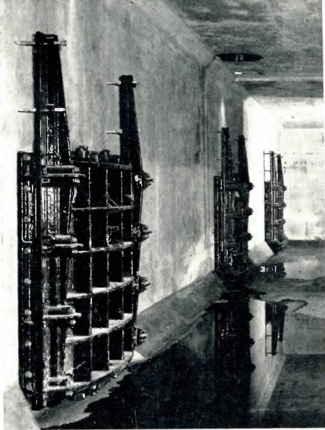
These are 60x60-inch discharge sluice gates from one of the three settling basins. The photograph was taken from the settled water header.
