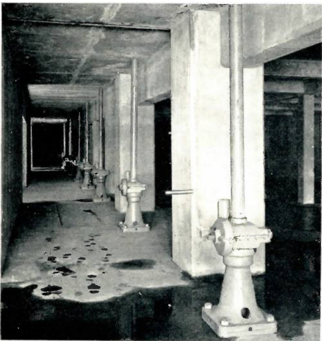
This bank of floor stands is for the manual operation of the 84x84-inch discharge sluice gates from the clear water header.
