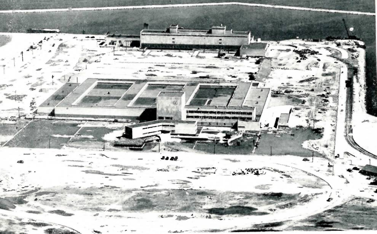
This aerial view of Chicago's South District Filtration Plant only partially indicates the size of the project. The structures of the plant cover twenty acres, eight of which are in buildings extending above the finished ground level. Part of the 2,700-foot rock-fill breakwater, which protects the project from wave action, is shown in the upper part of the photograph. Below is the Edward F. Dunne crib, located 3.2 miles off shore, one of the plant's two raw water intakes.
