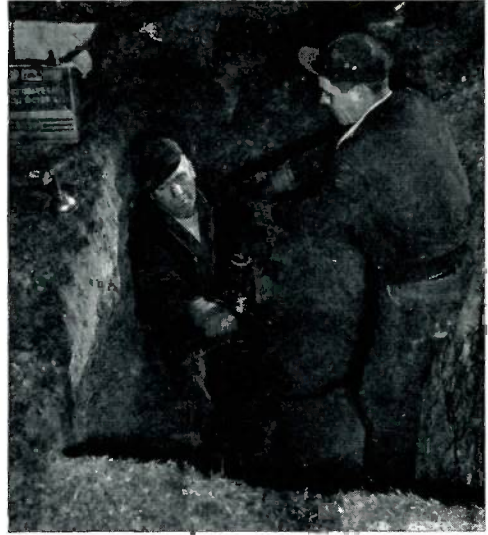
Willis Shumacher and Rodney Rohr tap a main under pressure with a Mueller A machine.
