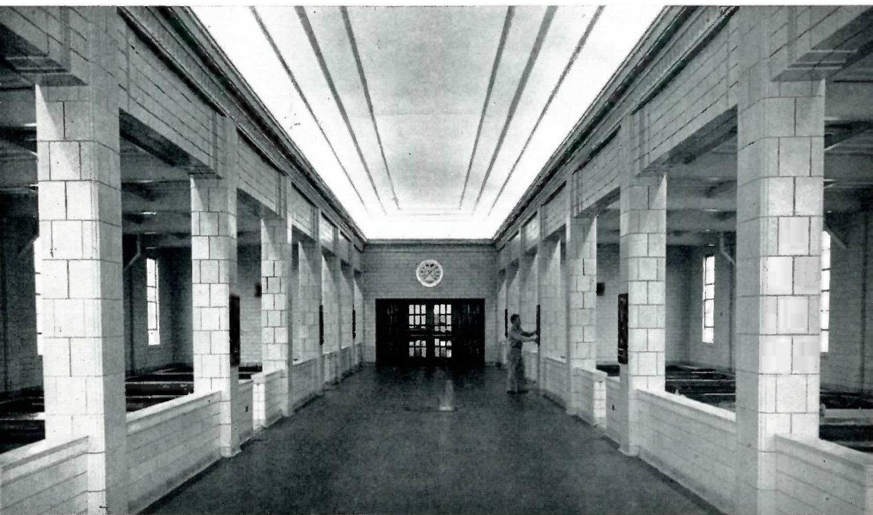
An interior view of the filter gallery. The filtration plant originally had four filters when it was built in 1936; four others were added in 1942. The operator shown in the photograph is M. Payne Gale.
