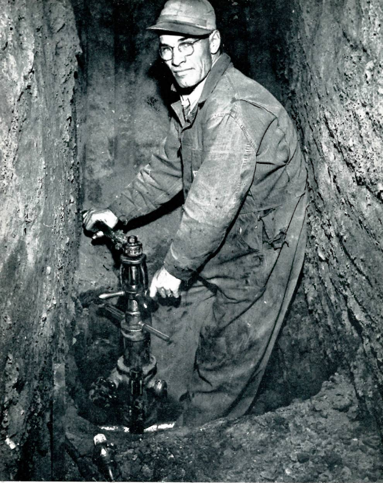
Adding a service connection to a Minot water main takes on the appearance of a major excavation project. Donald Mahoney, serviceman, is shown making a tap in a main, using a Mueller B machine.
