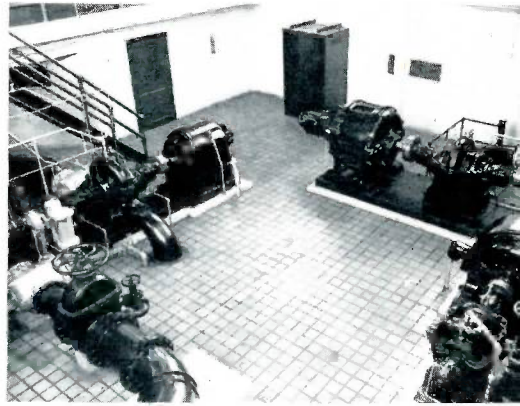
Pump Room, showing three of four units which comprise 21 million gallon station.
