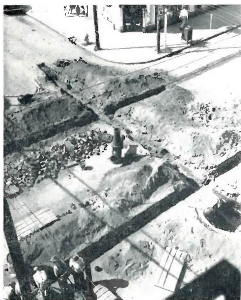
Busiest intersection downtown—Princess Anne and William streets—is criss-crossed with trenches as project is rushed across.
