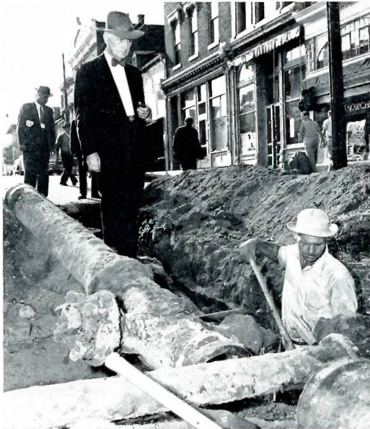
City Manager L. J. Houston, Jr., watches Fielding Coombs prepare ditch for new 16" C.I. water main. Pipe on bank was laid in 1884, and will be re-used in the gas and water distribution systems.
