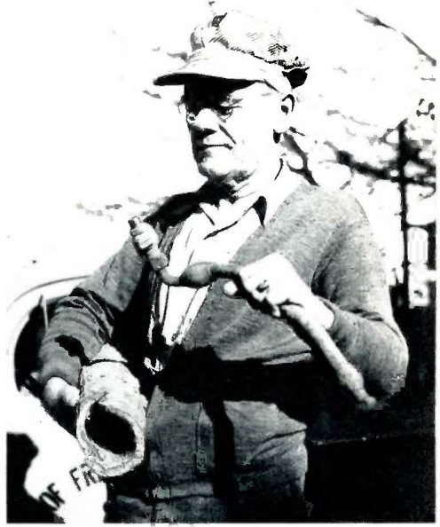
John L. Perry, Gen. Supt., holds a section of the old Aqueduct line laid in 1850. The stop and gooseneck are of 1884 vintage. Note varying thickness of iron in old pit-cast pipe.
