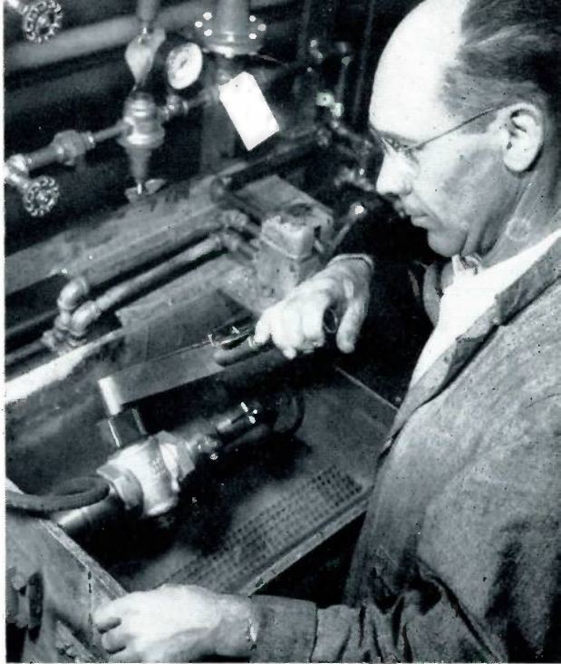
Engineer Wallace Gould intently observes the LubOseal stop while it undergoes severe testing. Gould did a major share of test work on the stop and made several suggestions which improved the new product. He learned that the LubOseal stop remained in practically the same condition after 1,000 operations.
