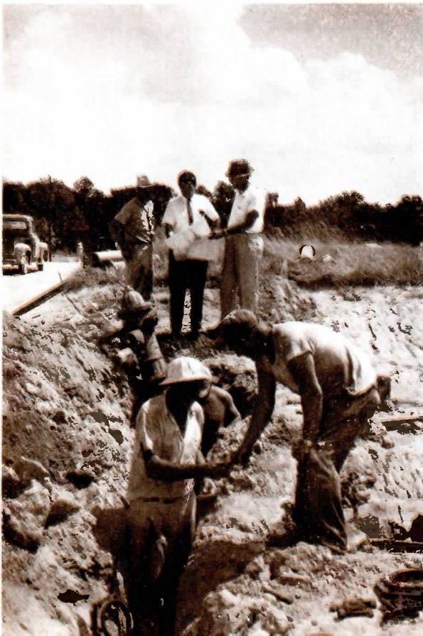
At the left, Nelson discusses progress on the water line work with Holloway of Holloway & Son and one of Holloway's men.
