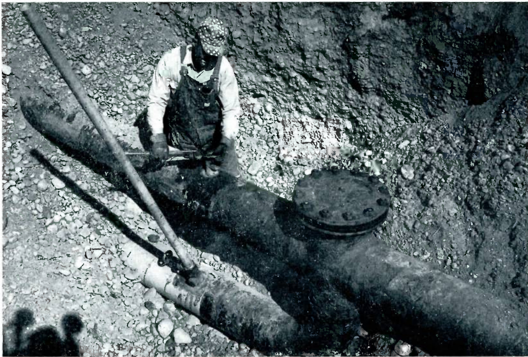
Watching the Mueller C1-36 drilling machine make its cut are, from left, Warren Crawford, Mueller's Western Section Manager; D. E. Stein, District Engineer for Washington State Highway Dept.; Walt Arnett, Mueller Sales Representative in the area; Elmer Young, Chief
