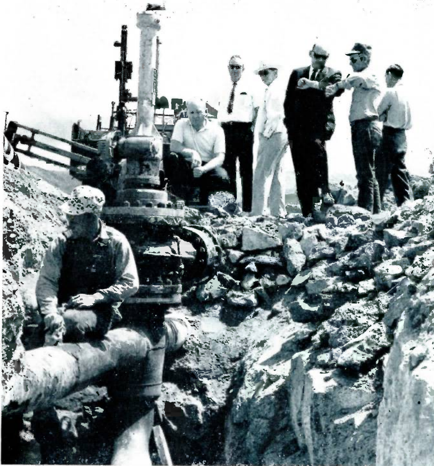
Checking progress on a line stopping job in Eastern Idaho are, from left: Jack Fouts, welder, Hood Corp.; Scott Busselle, Asst. Operation Manager, Intermountain Gas Co.; Charles Chesney, Operation Supervisor, Pocatello Division of Intermountain Gas; Mueller Sales Representative Walt Arnett; Ben Morache, Construction Supervisor from Intermountain Gas; Bob McAlister, Hood Corp. Foreman, and Lloyd Little, Operation Supervisor, Idaho Falls Division, Intermountain Gas. The new line can be seen coming out of the bottom of the fitting.
