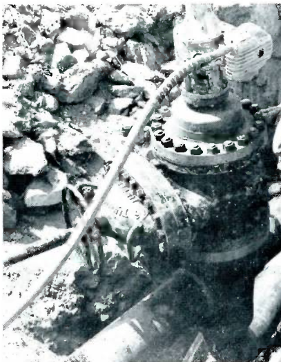
Gas Measurement Engineer Jerry McCormick checks a gate valve which will have a line stopper fitting bolted to it later. Below, the Mueller gate valve can be seen with the drilling machine attached.
