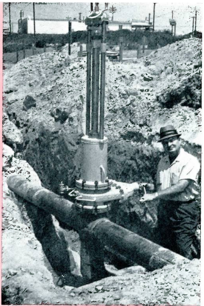
Shelby Gas Superintendent Jim Milsaps checks over a gate valve and Mueller line stopping equipment which were used to relocate the gas main without interrupting service along the line. Below, is the Mueller C1-36 drilling machine, its shell cutter and a section that was cut from the pipe.
