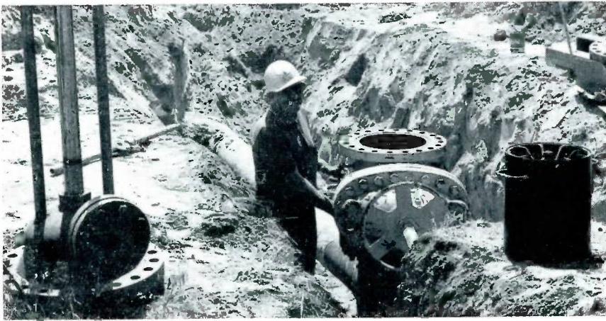
Gas Measurement Engineer Jerry McCormick checks a gate valve which will have a line stopper fitting bolted to it later. Below, the Mueller gate valve can be seen with the drilling machine attached.
