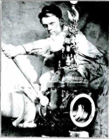
Herman Chepan of the Regulator Dept., tightening up a big gate valve.
