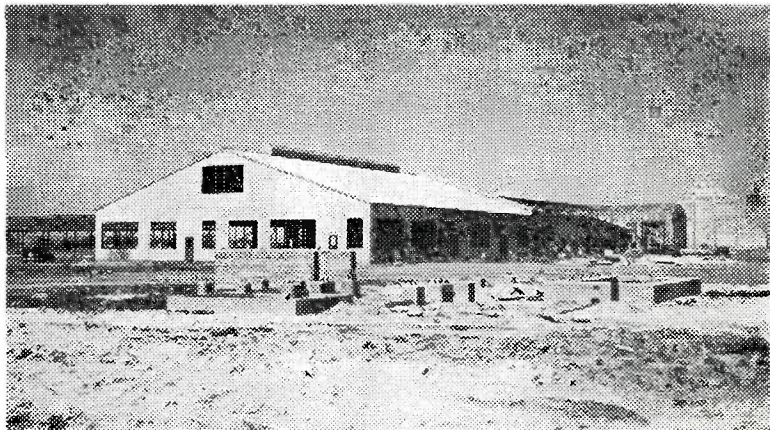
Top of page: Aerial view of elaborate layout of Western Cottonoil Co. At right: New compress building nearly completed.
