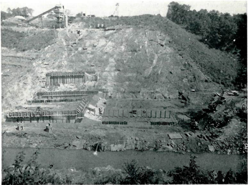
This photo shows the diversion of the Patapsco at the west side of the dam and the bottom concrete monoliths being poured.
