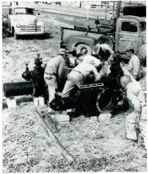
Workmen prepare the cross for hoisting into the hole. The 16-inch valve was needed in order that a new pipeline to the proposed new Caterpillar plant in Decatur might be laid.
