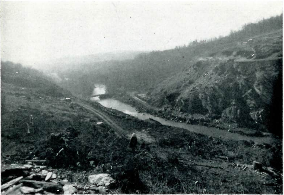
Here is a general view of the site that was cleared shortly after the contract was let. The temporary bridge over the Patapsco River can be seen in the distance.
