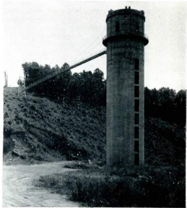
The 170-foot high intake control tower and its 270-foot aluminum suspension bridge is one and one-fourth miles upstream from Liberty Dam.
