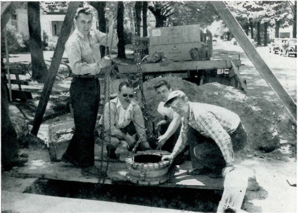
Shown lowering the slide valve are, from left, R. A. Martin of Battle Creek, superintendent of P & M Construction Company, Inc., Jack Rubicam of Grand Rapids, Mueller Co. sales representative, Peterson and Crowell.
