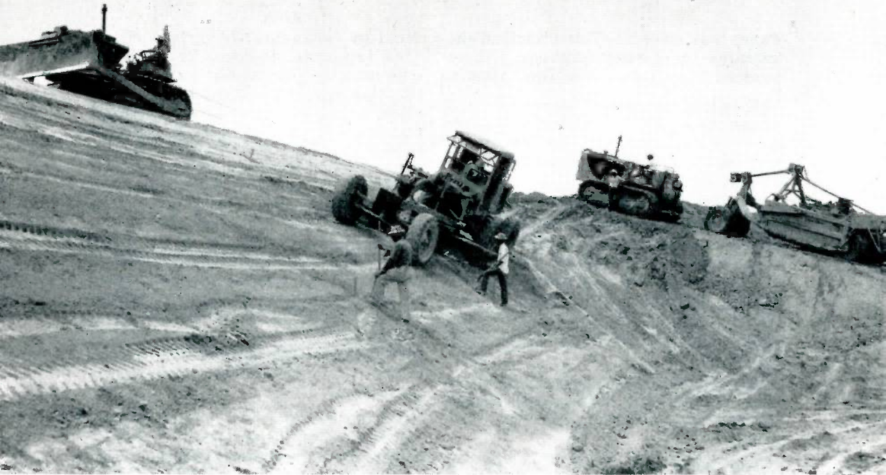
Earth moving equipment builds the circular pattern wall of Tucson, Arizona's new reservoir. Maximum depth of the water will be 24.83 feet. Diameter of the floor is 320 feet and the diameter of the roof is 414 feet.
