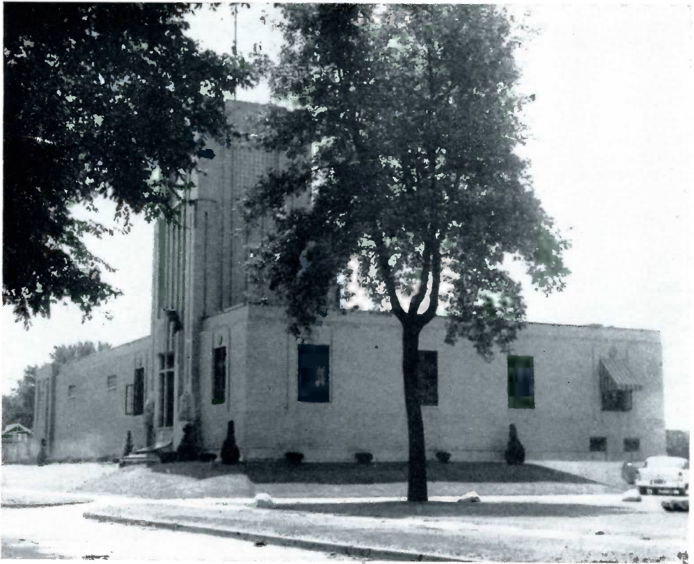
Looking at the softening plant from the west.
