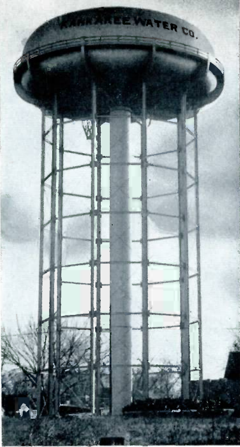
The 750,000 gallon elevated tank.
