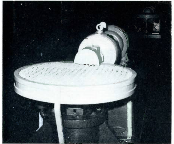
One of three chemical mixers at the Kankakee Water Company.
