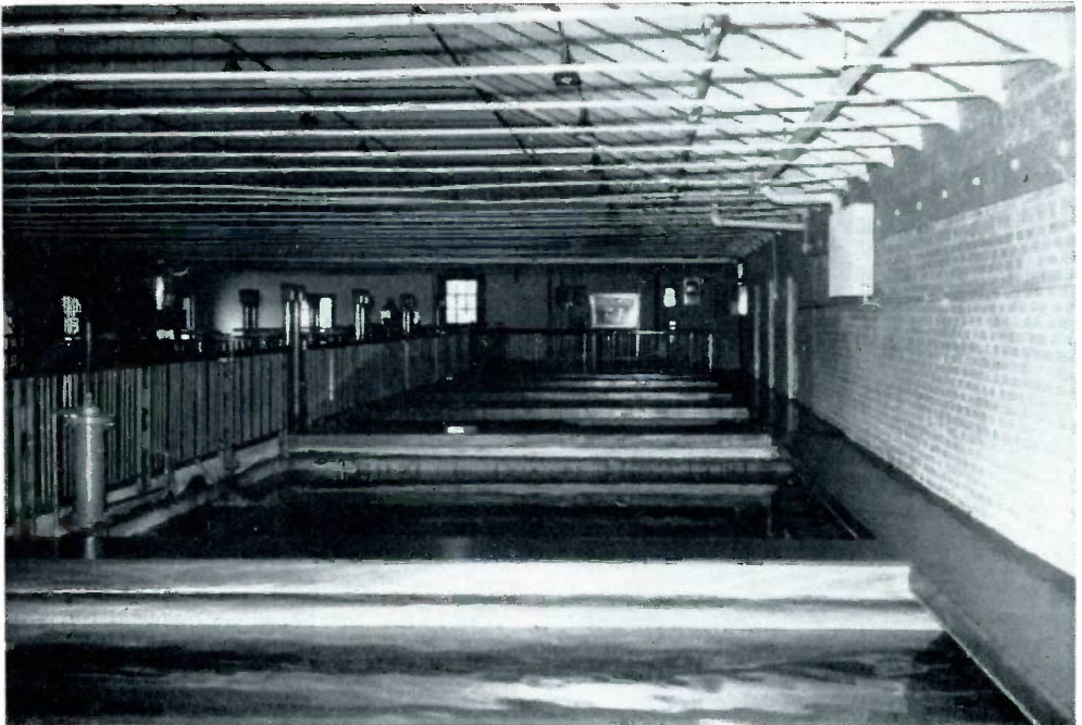
This view shows a part of the interior of the filter plant.
