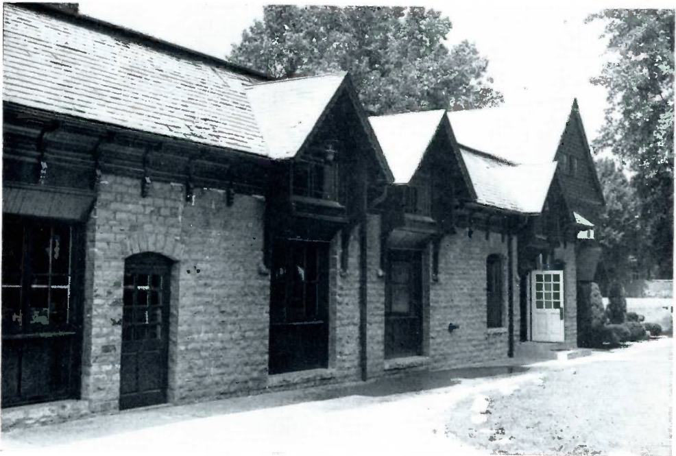
This attractive building is the Kankakee pumping station.
