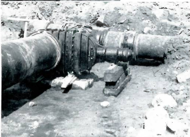
At the left is Ray Anderson, Superintendent in Pawtucket, Rhode Island. Below, a 24-inch Mueller valve is installed on the new line connecting a 24-inch force main to the new three million gallon tank, which you see in the photo at the right. Pawtucket has standardized on Mueller valves.
