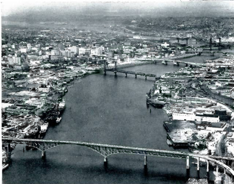
Another view of Portland, looking north along the River, showing the many dock facilities of this busy port.
