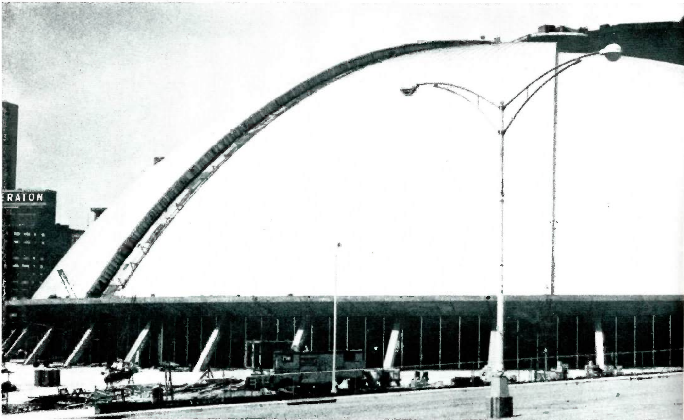
This dramatic view shows the huge metal arm which supports 190 tons of stainless steel in the dome of Pittsburgh's new auditorium.
