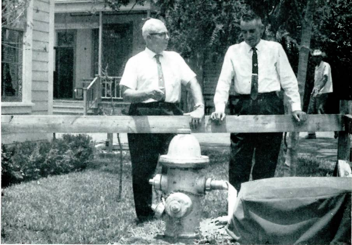
Above: Jack Cherry, Water Superintendent of Arlington, Texas (left) and J. D. Steadman, Water Superintendent of Grand Prairie, Texas, discuss installation of a hydrant on the grounds of SIX FLAGS.
