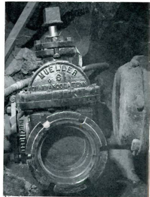
This closeup of a Mueller valve was taken after the drilling machine was removed and just before a piece of pipe was put in and the hydrant set.
