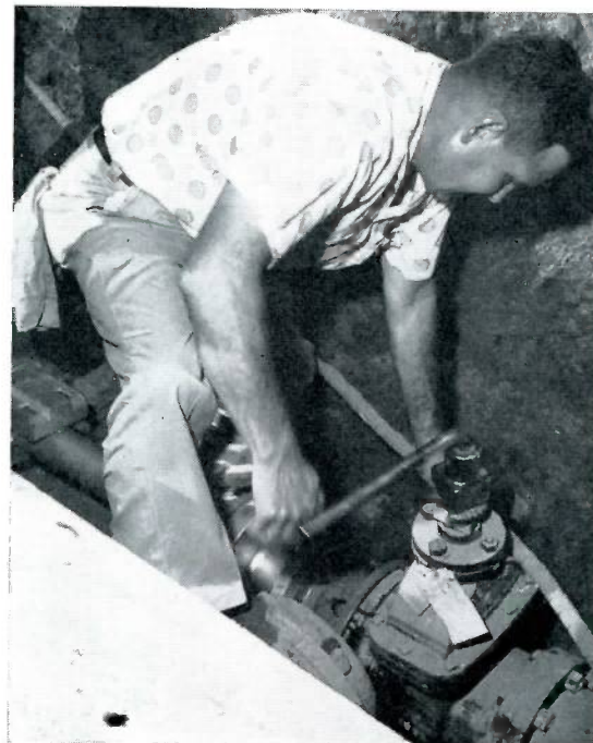
The gear drive box and flexible shaft on the gasoline engine drive unit are shown at left as the drilling operation begins (left). After the cut has been made, Mueller employee Lindle (Hap) Hockman closes the Mueller valve (above).
