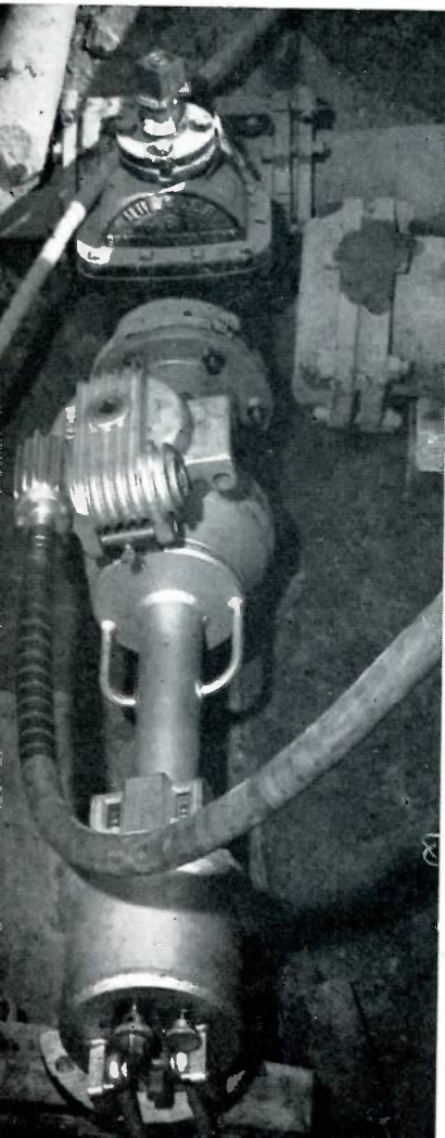
The gear drive box and flexible shaft on the gasoline engine drive unit are shown at left as the drilling operation begins (left). After the cut has been made, Mueller employee Lindle (Hap) Hockman closes the Mueller valve (above).
