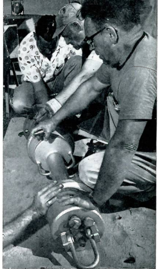
After the proper drilling equipment has been attached to the boring bar (above), a solid coating of Mueller cutting grease must be applied (right) to the shell cutter and pilot drill.
