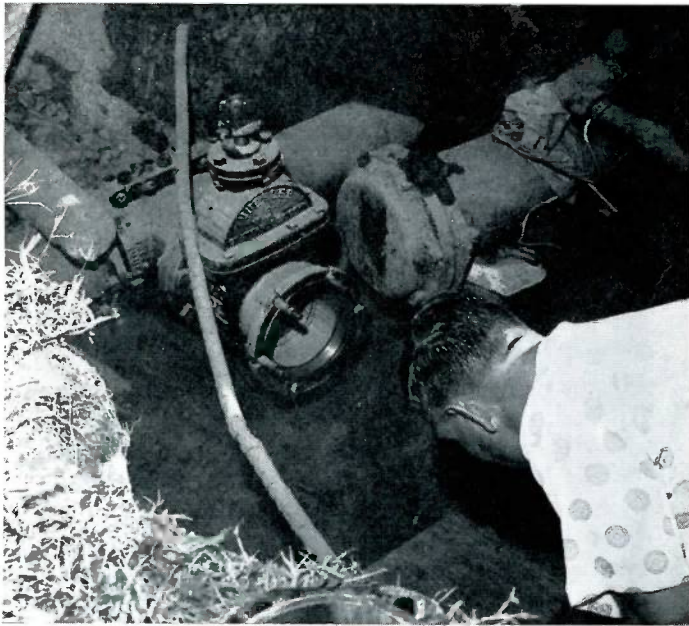
Unexpected obstacles often are found when excavations begin, and this job was no exception. The Mueller Tapping Sleeve and Tapping Valve are shown amid pipes and cables.
