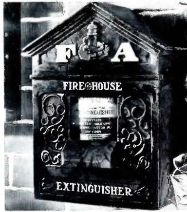
This old-fashioned fire alarm box doubles as a fire extinguisher cabinet.
