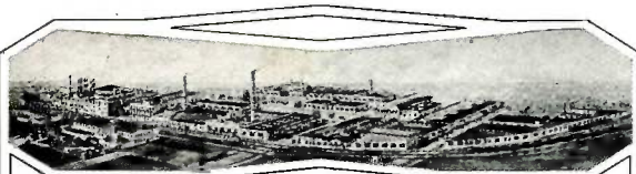
MAIN PLANT Decatur, Ill.
