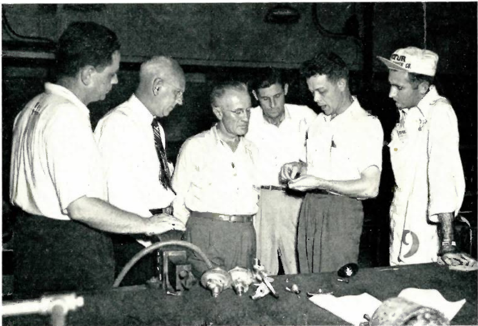
Loren Grosboll, second from right, regulator engineer, demonstrates the Mueller-patented auxiliary spring principle of a relief valve to George Knipe, J. L. Logsdon, Paul Hines, Harold Linton and A. D. Parks.
