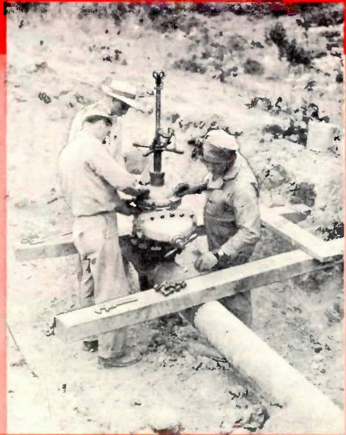
Third phase of the job with Mueller equipment is the use of the completion machine.
