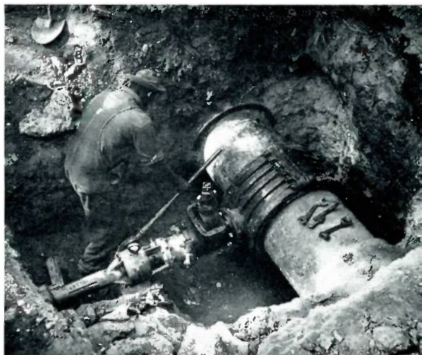
A Mueller C-C drilling machine and tapping sleeve and valve are being used to cut a 24-inch main for a fire hydrant installation.
