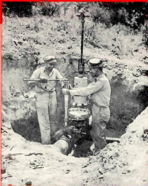
Tapping the line with a Mueller D.4 drilling machine to empty the line of gasoline.
