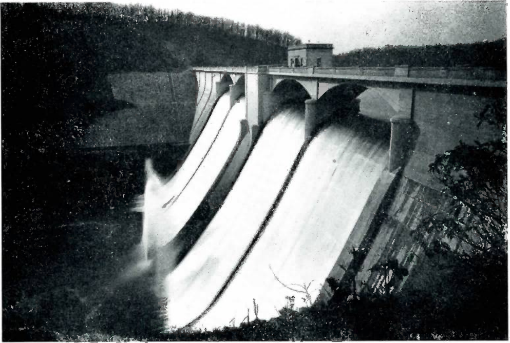
This dam on the Prettyboy branch of the Gunpowder Falls impounds 20 billion gallons of water. The four spillways total 274 feet in length and rise 130 feet above the stream bed. Prettyboy dam was completed in 1933. It is 25 miles upstream from Loch Raven dam.
