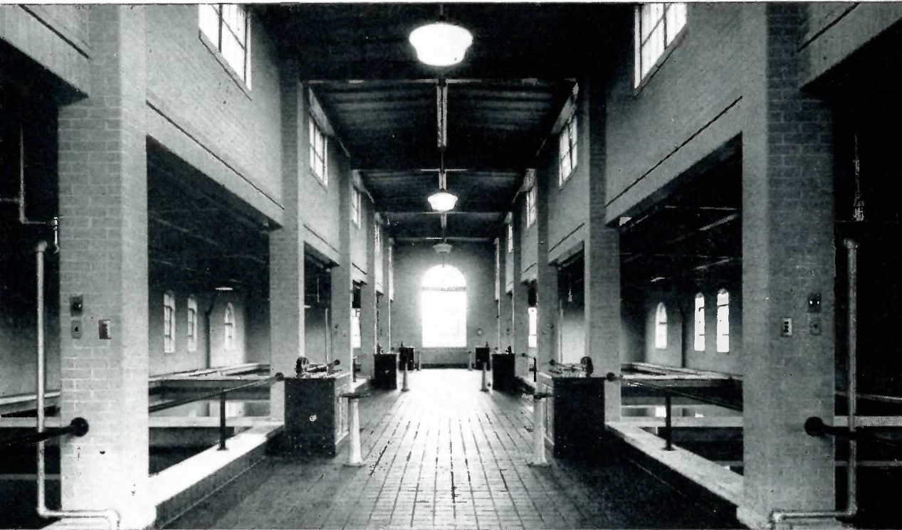
An interior view of the City Water Company's No. 3 filter building. Chattanooga, Mr. Porzelius points out, was one of the first cities in the South to have been provided with filtered water.
