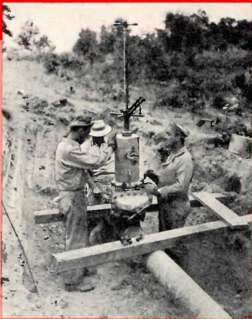
Next the stopping machine is bolted on and the stopper seated, halting the line's flow.
