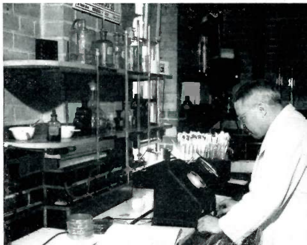
Quality of Chattanooga's water is carefully controlled through laboratory tests. Here C. V. Swearingen makes a bacterial plate count.
