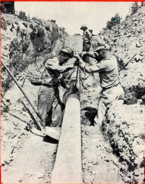
With the flow stopped and the line empty, a pipe cutter is used to sever the line.
