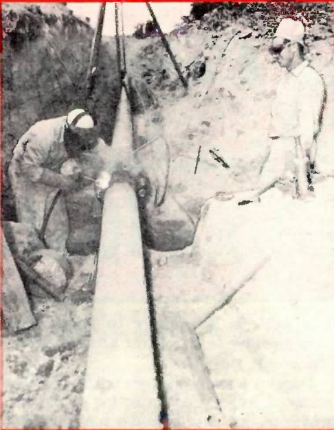
The insulating flanges are then welded into place, isolating the crossing electrically.
