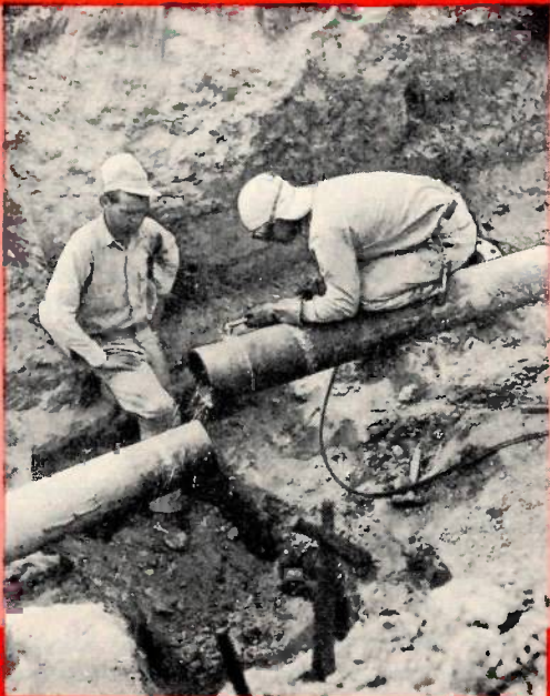
An oxy-acetylene torch is used to cut away a small section of the line for the flanges.
