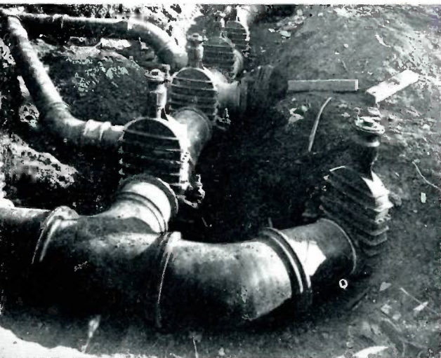
This is a view of an installation of Mueller Co. gate valves at the 30-inch low header discharge of the Citico Pump Station.
