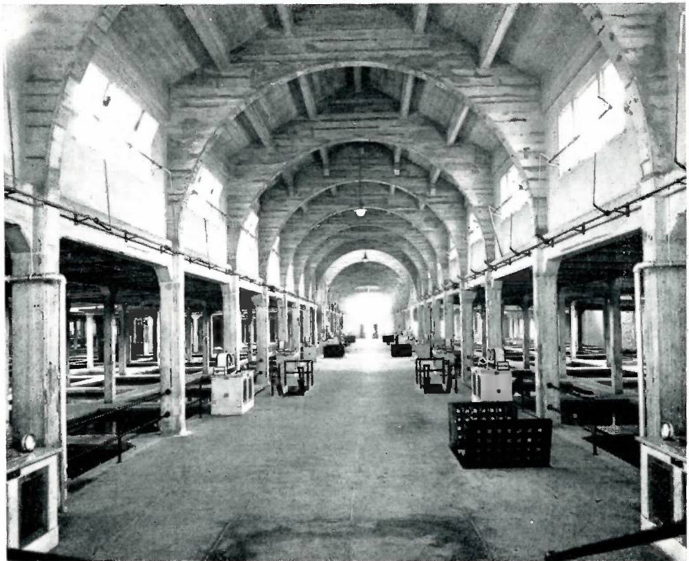
Interior view of filter gallery in plant No. 1, showing the filter units and control tables.
