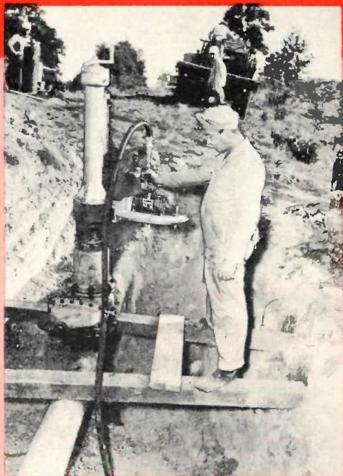
A Mueller C-1 machine cuts into the Phillips line on the upstream side of river crossing.
