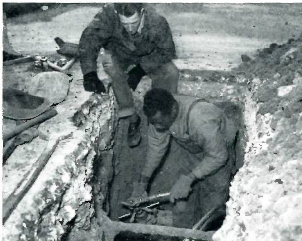
Foreman Bill Evans and Serviceman Percy Rawls making a tap in a 6-inch cast iron main, using a Mueller B tapping machine.
