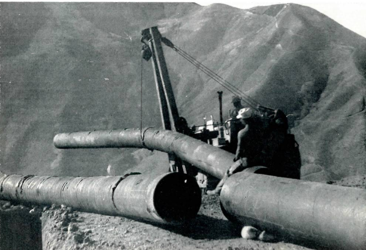
Figure II. Handling one of the bends with a sidearm Caterpillar. Rough terrain made operations difficult in this area.
