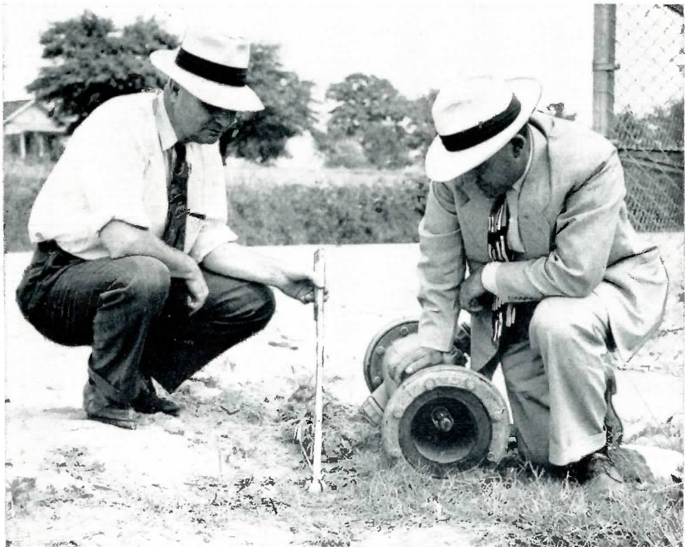
L. E. Wallis (left), Elberton Water Superintendent, and M. M. Chapman (right), representative of Grinnell Co. of Atlanta, Georgia, inspect the safety thimble which opened automatically when the hydrant barrel was knocked over.
