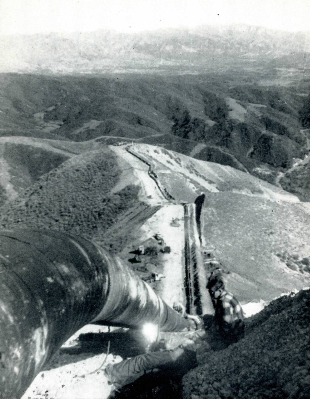
Figure III. Tying in the pipe preparatory to lowering in the trench. Note the crooked, uneven right-of-way which hampered operations.
