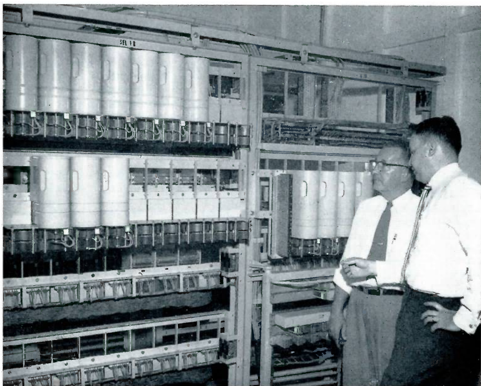
What makes our inter-plant dial telephone system function is explained to E. F. Dickey, office manager, by Tommy V. Atkins, service engineer for the Illinois Bell Telephone Company. Mr. Atkins is located in the company's Decatur office and was instrumental in our change from the manual to the dial system.
