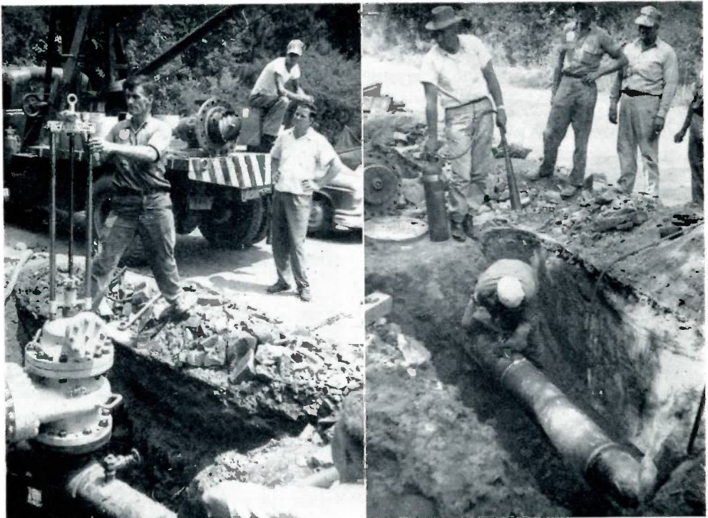
The stopper is set in the fitting and is being expanded in the photo at left. Note the section of pipe removed from the line to accommodate the stopper retained in the shell. At right you see the cutting of the line to permit installation of the plug valve at Charlotte. This permits the removal of the line stopper equipment.
