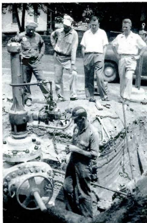
A Mueller C-1 air power operated drilling machine is making cut in ten-inch Mueller line stopper fitting. In background at right are A. D. Parks, Southeast sales manager, and Lorin Grosboll, sales representative for Mueller Co. Other three men are Piedmont Natural Gas Company employees.
