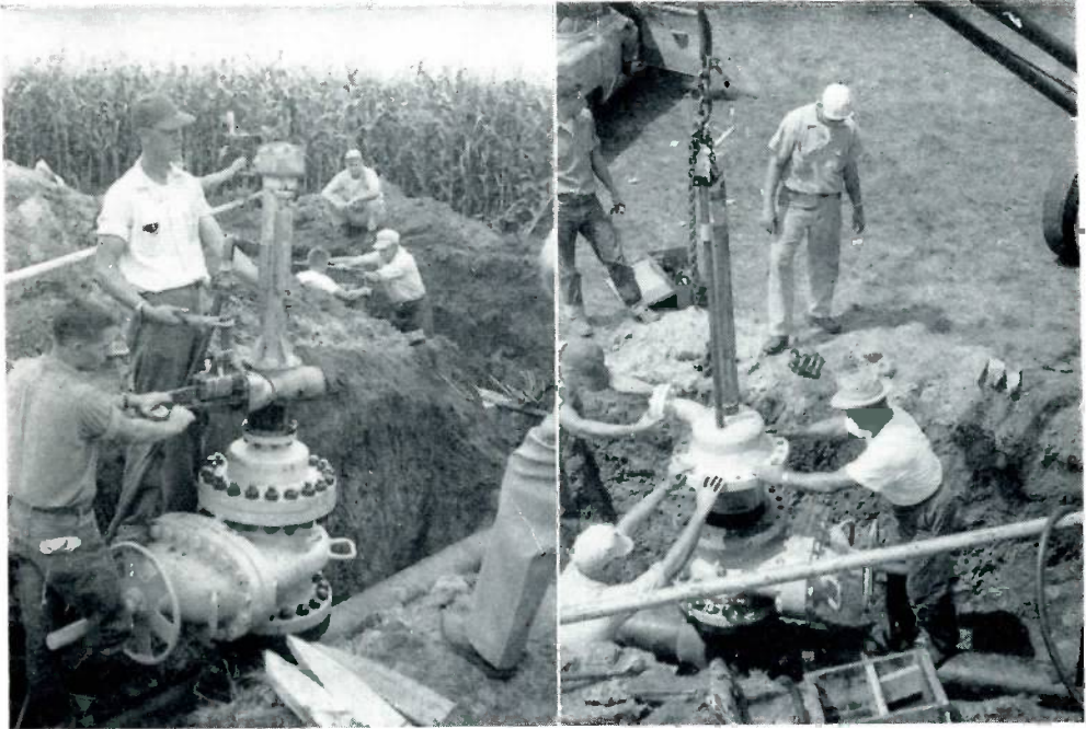
At Tuscola, Illinois, Panhandle Eastern Pipe Line Company workmen use a Mueller C-1 drilling machine in the photo at left to make a cut in the Mueller ten-inch line stopper fitting. At right, workmen are attaching the steel wedge stopping machine to the gate valve.
