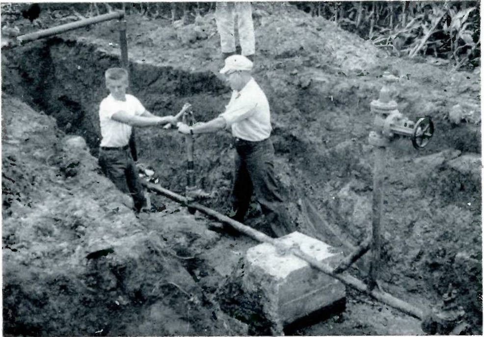
Panhandle workmen use a Mueller D-4 drilling machine in order to drill this two-inch line stopper fitting.
