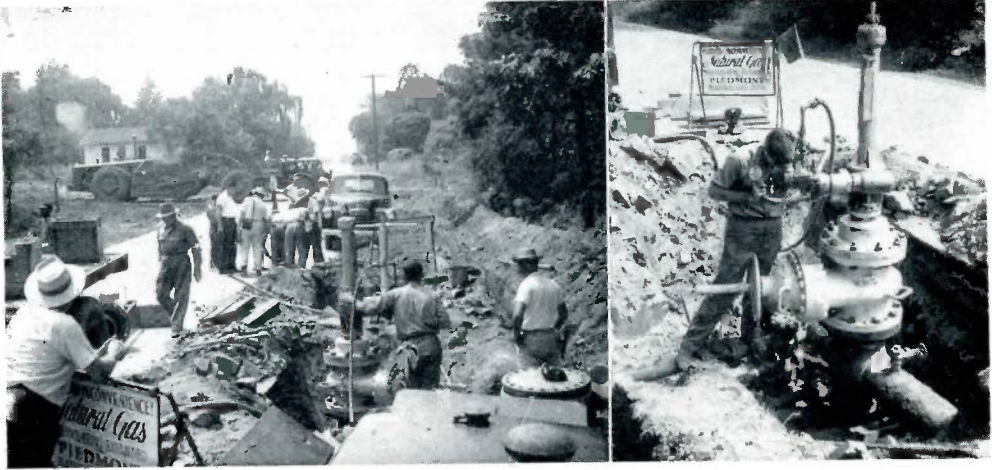
At left is a general view of the operation near Charlotte, North Carolina. One fitting is in the foreground where a C-1 drilling machine is in use. The truck in the rear is the location of the second fitting. Rock had to be blasted to lower gas main. The photo at right is a close up of the drilling operation as shown in the general view.
