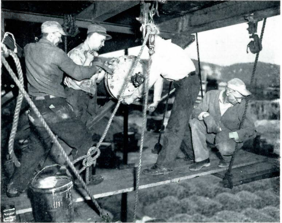
Under difficult working conditions, Equitable distribution crewmen cap the open end of a 16" line which is being cut off. This particular line, strung along the underside of one of Pittsburgh's 148 bridges, was dismantled to facilitate construction of Pittsburgh's new Penn-Lincoln Parkway, a 27 mile expressway that will speed east-west traffic uninterruptedly across the heart of the city.
