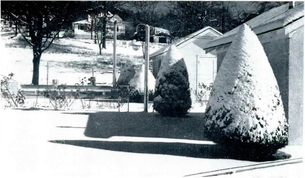
Partial view of Arkansas Western Gas Company's Fayetteville Border Station on a cold winter day.
