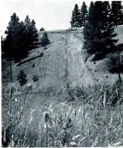
THESE TWO SCENES are typical of the path followed by Montana Power Company workmen in laying natural gas mains to Missoula. Locations of the main is shown by the freshly covered earth forming a pathway.
