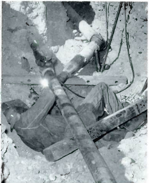
A MONTANA POWER COMPANY welder, at right, welds a Mueller line stopper fitting to the line that will increase delivery of natural gas to a chemical company near Butte. At left, William E. Blackman, Montana Power Company foreman in charge of the project, and Mueller Co. sales representative F. R. Seevers, observe the operation.
