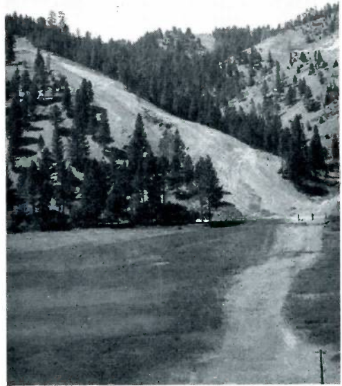
THESE TWO SCENES are typical of the path followed by Montana Power Company workmen in laying natural gas mains to Missoula. Locations of the main is shown by the freshly covered earth forming a pathway.
