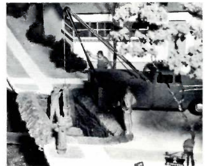
A Mueller "C" Machine is lowered into position to install an inserting valve in front of the Smith's.
