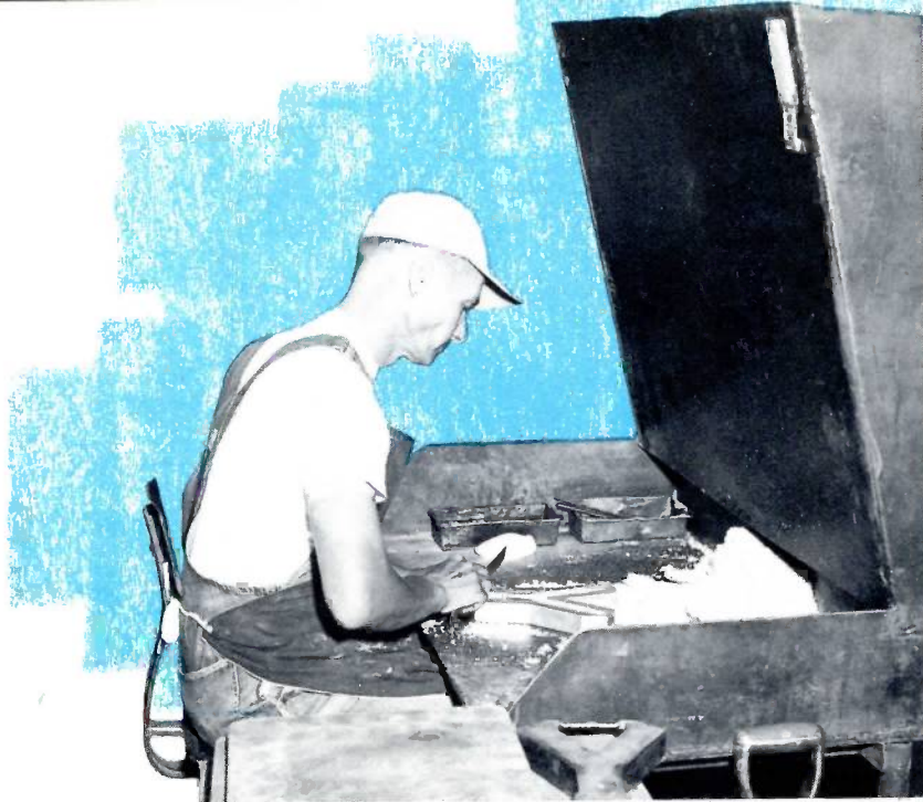
Skilled hands of expert coremen utilize long experience, craftsmanship and unerring skill in shaping cores to exacting detail, even to the grain of sand.
