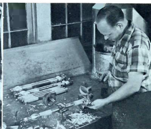
A steady hand and a "fire-proof" thumb are the necessary tools of this skilled workman as he "wipes" a lead gooseneck joint to mirror-smooth perfection.
