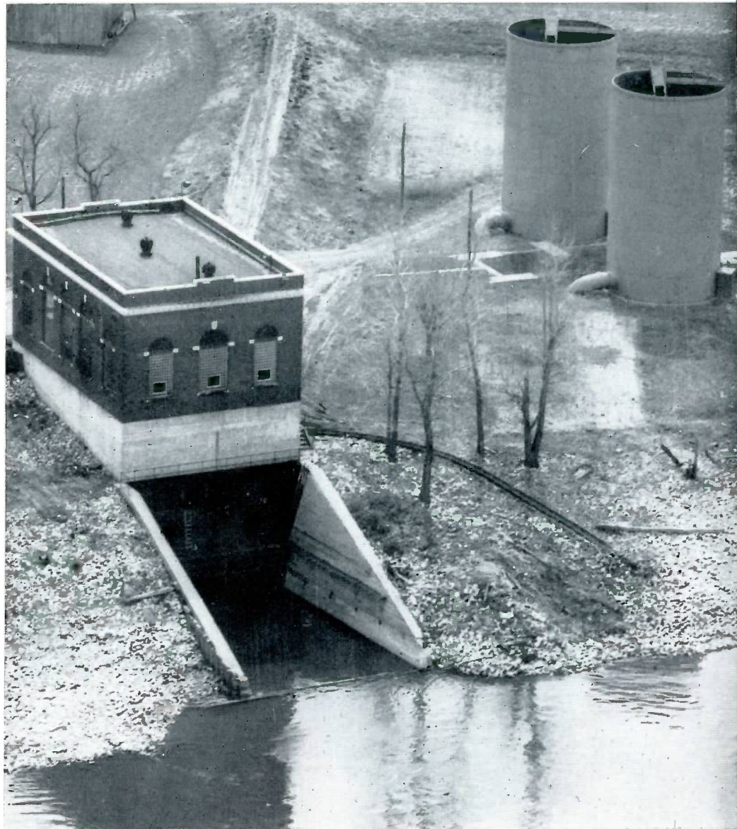
Aerial view of Chouteau plant, where a 30-million-gallon pump elevates water ninety feet into the two storage tanks seen at the upper-right.
