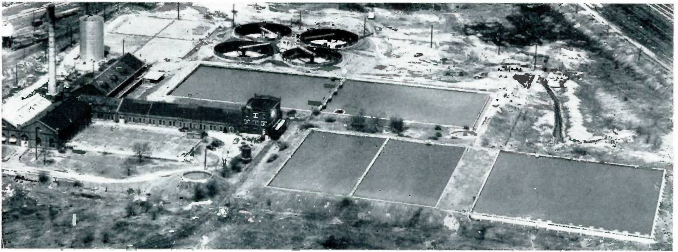
Aerial view of main pumping and purification plant at East St. Louis. In the upper background, four circular filters near completion. They added ten million gallons
