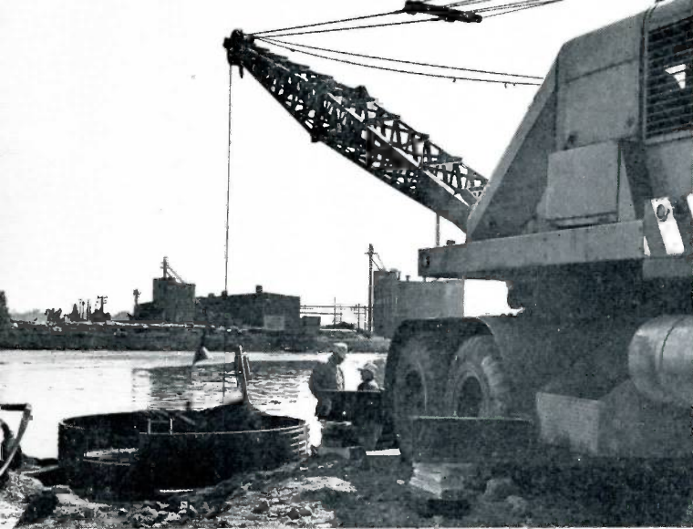
The shafts of the tunnel under the Calumet River are concrete lined within steel forms as shown here. The shaft is nine-feet in diameter.
