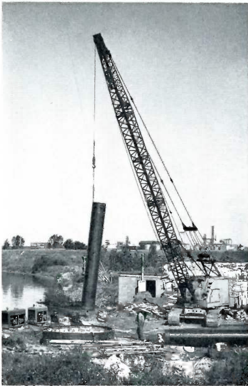
Twenty-foot lengths of 30-inch steel pipe, weighing about 1\frac{1}{4} tons were lowered into the shaft by a dragline. The pipe normally is shipped in 40-foot lengths, but had to be cut on the job so it could be lowered and maneuvered into place and turned at the bottom of the tunnel shaft.
