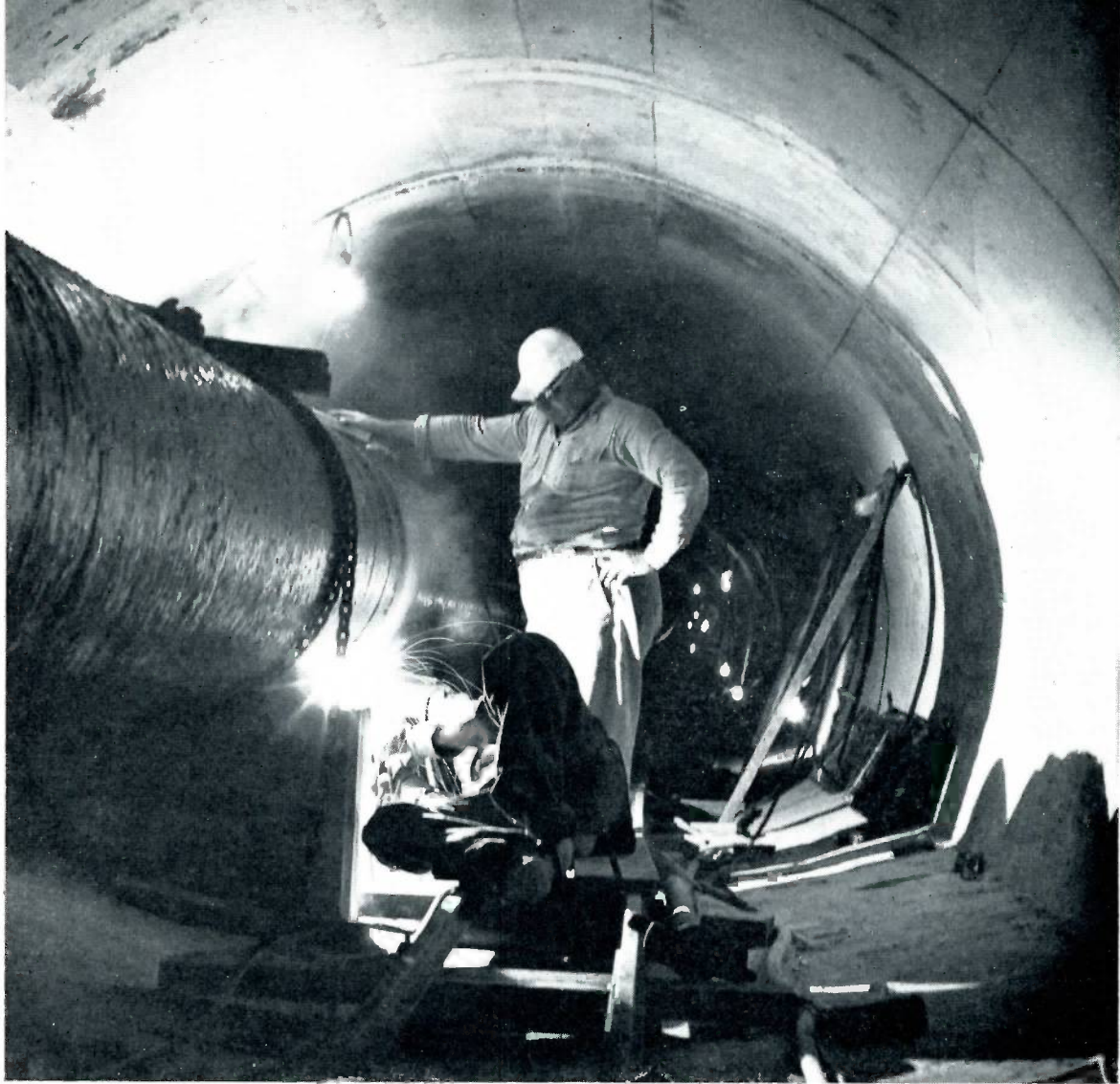
The steel 30-inch gas pipeline in the tunnel was welded in place after being moved to its proper location on small track cars. The track was removed after the tunnel was completed by the contractor. The estimated cost of the tunnel was placed at $481,000.
