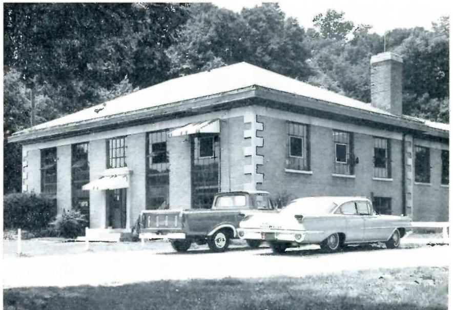
The original Griffey Lake Treatment Plant (above) has a filtration capacity of three million gallons daily. To meet increased demands for water, a large addition was started in 1954, providing total facilities which are capable of treating 7½ million gallons daily.
