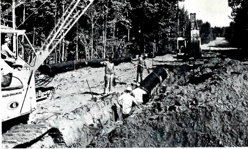
Workmen running a 36-inch collector line from the well loop to Alexandria's storage tanks.
