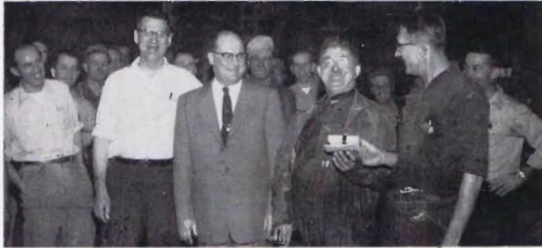
The above two photos were taken just at the climax of the careers of two long-time Mueller Co. employees. In the upper photo, Leroy Stout who spent twenty-nine years in the brass foundry, accepts a wrist watch from Roy Woods, brass foundry production control manager, on behalf of fellow employees. Looking on are Clarence C. Roarick, vice president in charge of Decatur factories, Leland Hartwick, brass foundry foreman, and members of the foundry who worked with Mr. Stout. The bottom photo shows Paul H. Jeschawitz proudly receiving a Hamilton pocket watch from Pete Kelley, Department 37 Steward. August Rauschek, foreman of Machine Repair, Mr. Roarick and members of Machine Repair Department look on.
