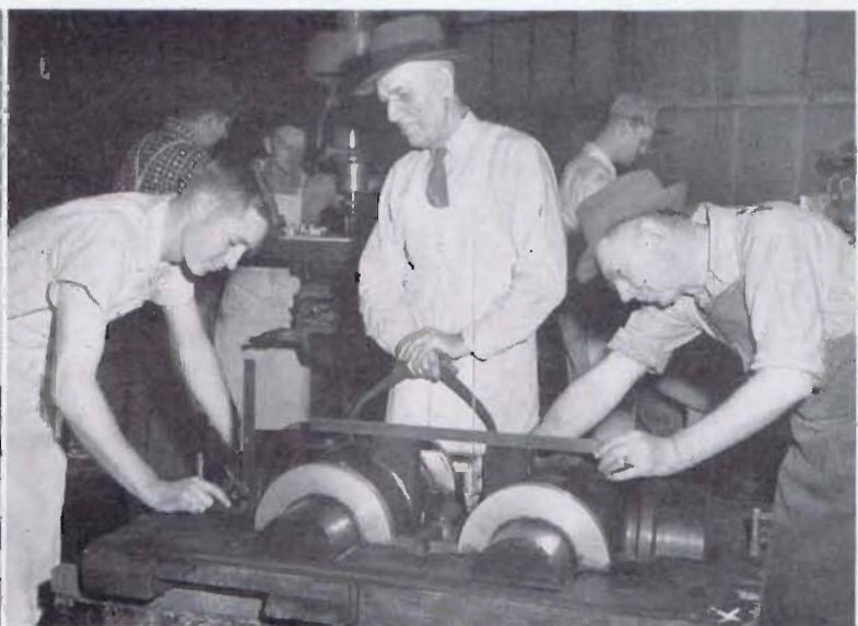
The pattern and core box are taken from storage, checked and issued to the Core Room by the Pattern Shop. The picture at the right shows Billy Andrews, left, and Roy Smith, right, checking the pattern under the supervision of Hugh Churchill, Pattern Shop foreman. In the foreground, three other pattern makers are at work. They are, left to right, Dick Anderson, John Graves and John Howard.
