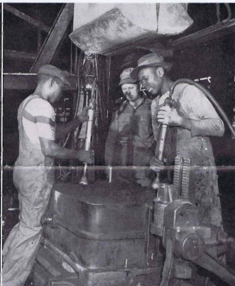
machine. Also shown is the half that they have just finished. At right, three 4,000 pound Herman Rollover machines are shown with two molders butting off the cope of the mold. Molders are Charley Kyle, left, and Clifford Thorton, right, with Group Leader Au'ta Fant looking on.
