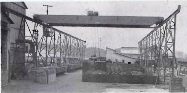
Here is our new Crane Way, most recent addition in the expansion program at our Chattanooga plant. The Crane Way has an 80-foot span and rises 35 feet from the ground to the top rail.
