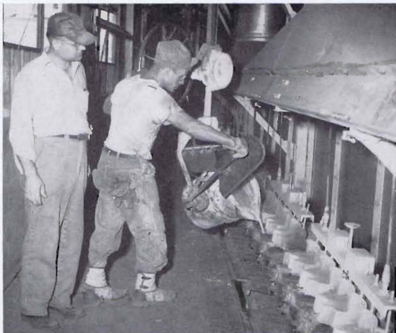
At left, Leland Hartwig, Brass Foundry foreman, observes Clarence Albert, ladleman, pour molten brass into a train of molds shortly after they were made by the machine molders. The train is in the pouring zone. Note the mold weights which are automatically lowered onto the mold to prevent metal from leaking out. After pouring, the train leaves this section and is pulled to the cooling site before being dumped. Once molds are dumped, the castings are separated from the sand by a Simplicity Shakeout which is a large vibrating machine that allows sand to go through it down on a belt conveyor. Castings go from the shakeout onto a metal conveyor where they are removed and stacked on skids
