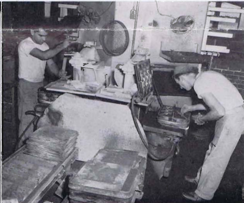
Hattie Zylicz, in foreground, and Bramlette Johnson are cleaning and inspecting cores before they go to molders. Both ladies have been with Mueller Co. eleven years. Center, Ramon Ballesteros is peening a mold. Vance Ziebarth, a twenty-year employee, at right, is
