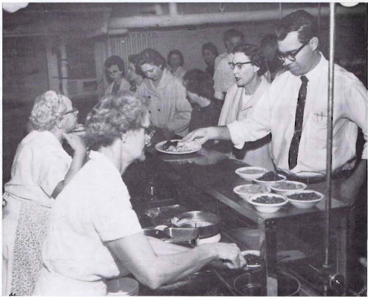
EMPLOYEES PASS THROUGH SERVING LINE
