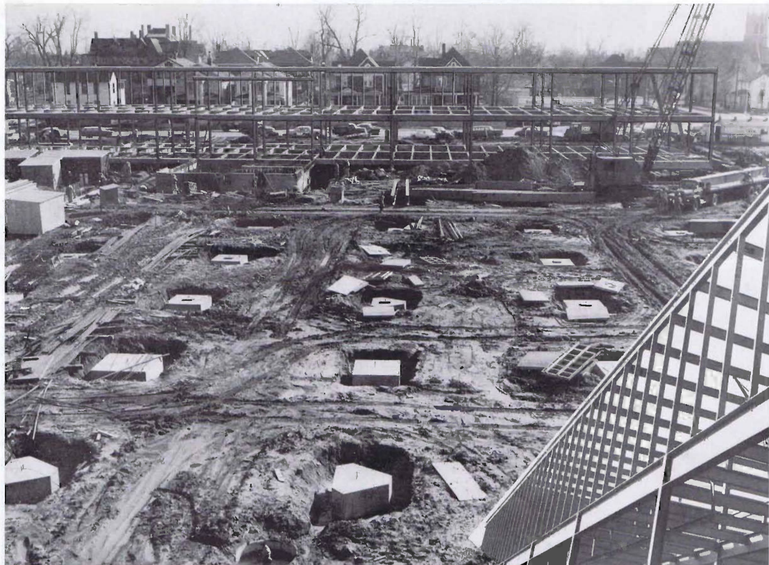
The structural steel for the new office building in Decatur is shown in the background while in the foreground are the capped piling for the support of the steel columns. The varying shapes of the caps are due to the number of piling in each cluster. The number of piling is
