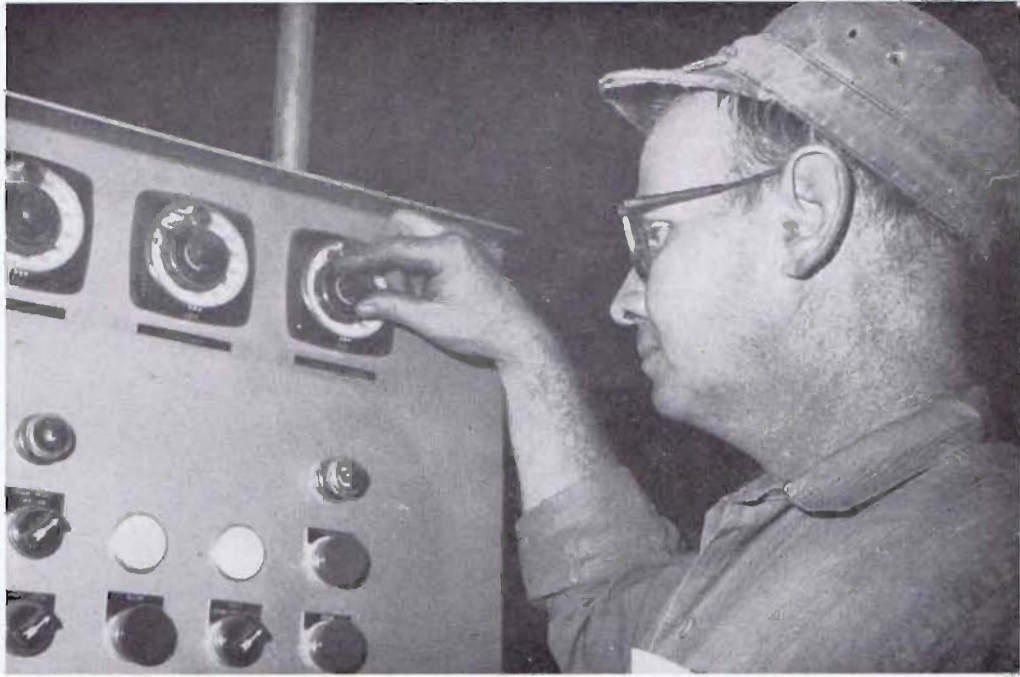
Here, Ray Edwards, Shell Core Set-Up Man, checks one of the many panels of dials, lights and other indicators that are necessary for the operation of the plant.
