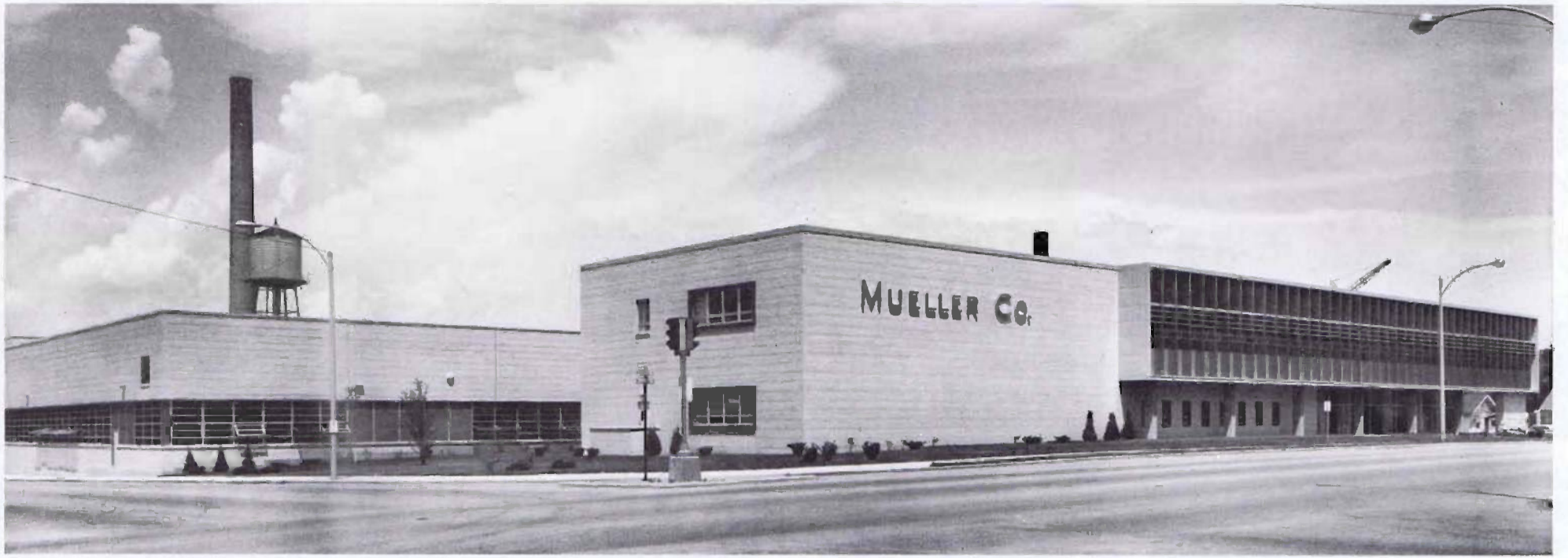
The completed office (right) and warehouse. The final portion of the expansion project in Decatur is expected to be finished by spring. Workmen are now laying brick, and
