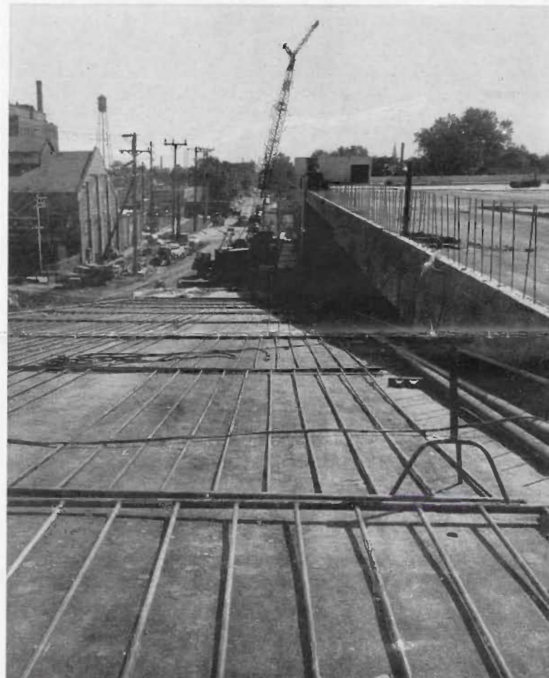
Trucks hauling Mueller Co. products, rather than construction trucks, are now using this area as Mueller Co. recently began using the new shipping dock which is shown at the right. A portion of the ramp leading to the roof-top parking is shown at the left and below. This network of pipes (below) is now covered by concrete and in a few weeks employees will be able to park on the roof. About 1.75 miles of pipe are included in the system to keep snow and ice off the ramp.
