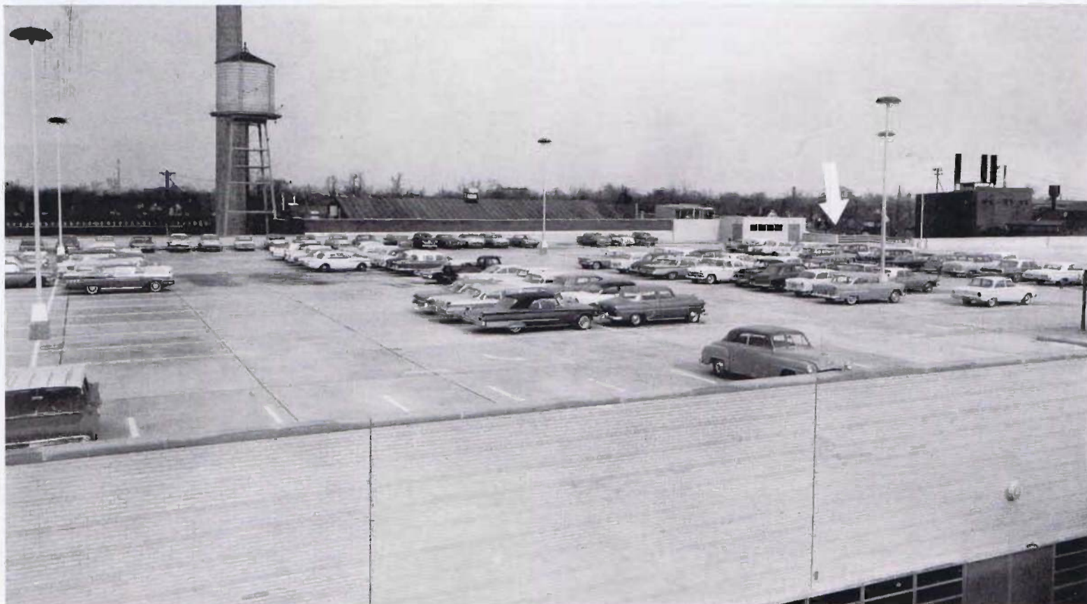
A portion of the 4½-acre rooftop parking area is shown above. The white arrow on the right shows where the ramp is located. Just to the left of the ramp is an employee entrance to the plant. At the
