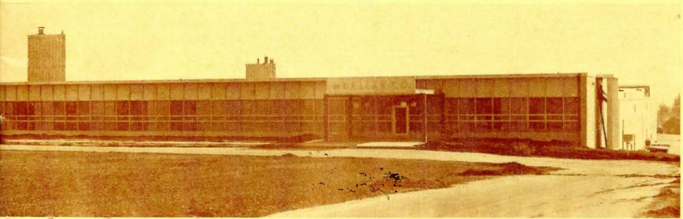
The office building's facade features special panels set in aluminum frames, and glass. At the far left can be seen the brick wall around the patio which is just outside the
