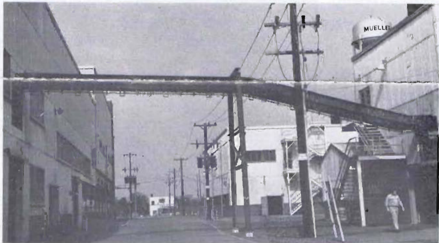
This overhead conveyor carries finished gate valves from the assembly and painting area (left) to the warehouse at the right. This street runs between the main manufacturing buildings on the left and the warehouse and shipping facilities on the right.
