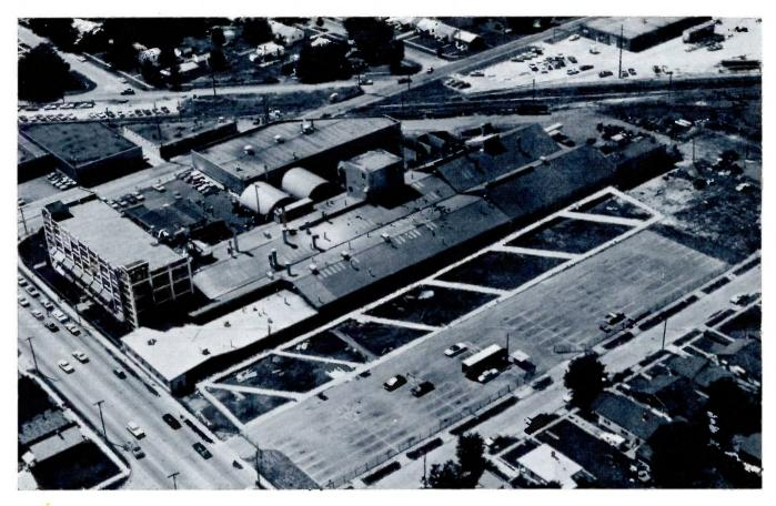
The 70-foot by 480-foot expansion at the Decotur foundry is outlined by the white lines. On the upper right end of the expanded area a new shipping and receiving dock will be added. The building on the lower left, currently housing core storage, will undergo major changes also during the program. The south wall will be
