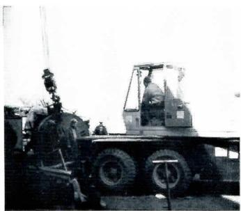
Linemelt furnace being moved into place and muller being lowered through the roof and put into place makes the Iron Foundry take on a new face.
