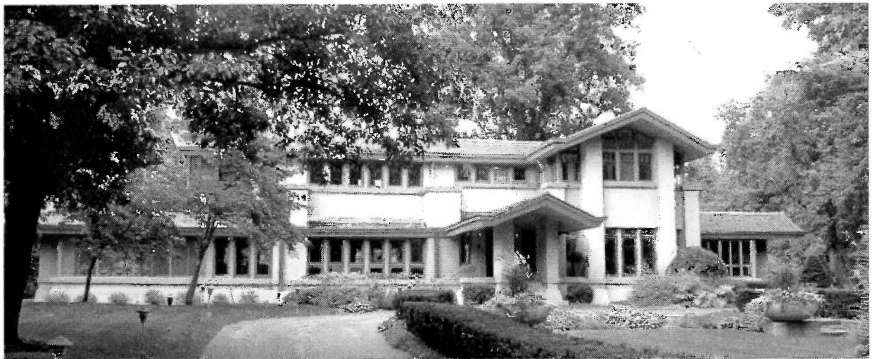
#4 Millikin Place – Adolph Mueller Residence
